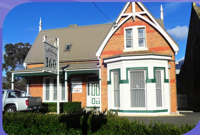
The Old Parsonage, 160 New Town Road, New Town
